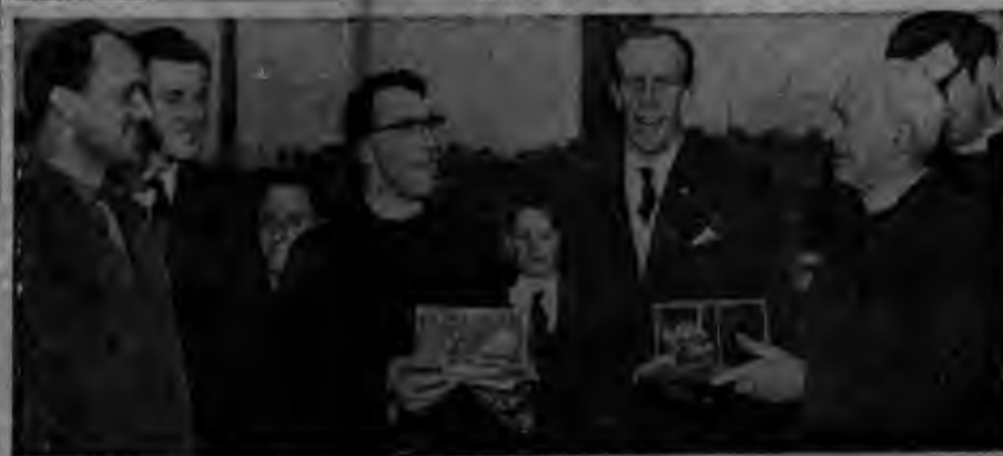
Canon A. M. Cook, using a Ruston-Bucyrus excavator, cuts the first sod on the site of the new St. John's (Ermine) church after a thanksgiving service last night. Below: Canon Cook (right) and Rev. J. Hodgkinson look at the model excavators that Mr. P. G. Hodgkinson (joint manager-director of Simons Ltd.) (centre) presented to them after Canon Cook had cut the first sod.
